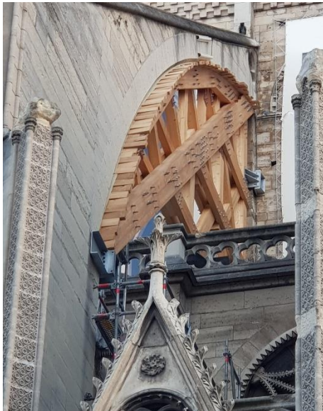
Figure 12: Consolidation of flying buttresses, August 2019 – Image Kai Weise
