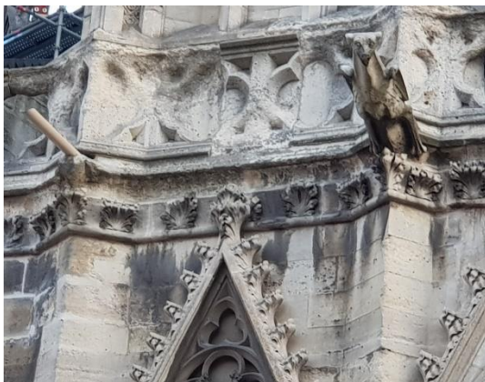
Figure 6: Missing gargoyles and deteriorated stonework - image Kai Weise
