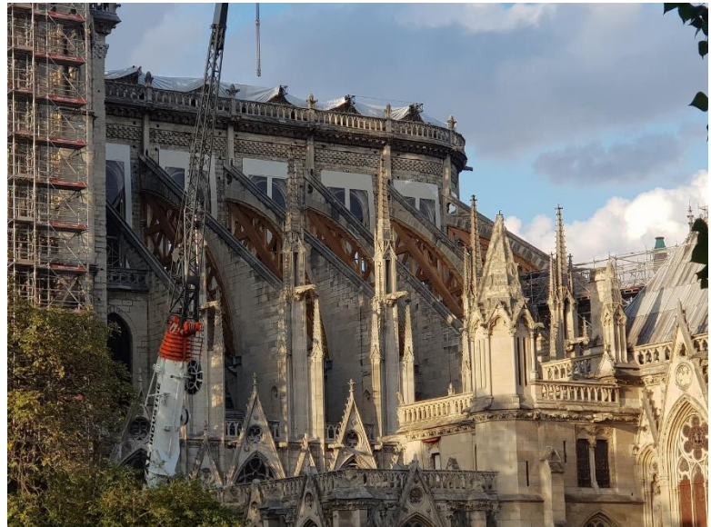
Figure 13: Consolidation of flying buttresses, August 2019 – Image Kai Weise
